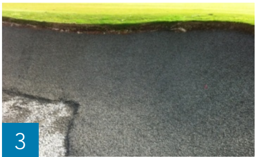
Spread Capillary Concrete at 2 inches (50mm) uniform thickness
